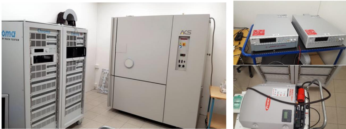
Fig. 2. The Energy Storage Laboratory
