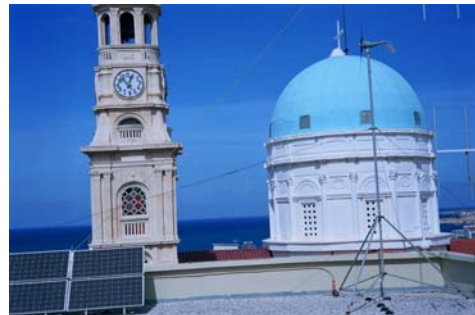
The RES installations(PV and W/T) on the roof of the Lab
